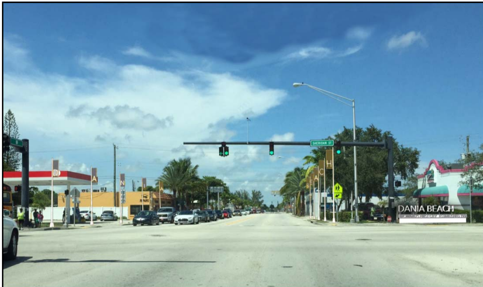
Northbound at Intersection of US1 and Sheridan Street: Option "B"
