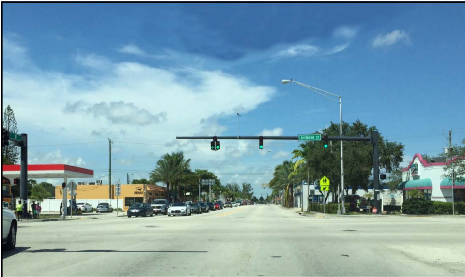
Northbound at Intersection of US1 and Sheridan Street
